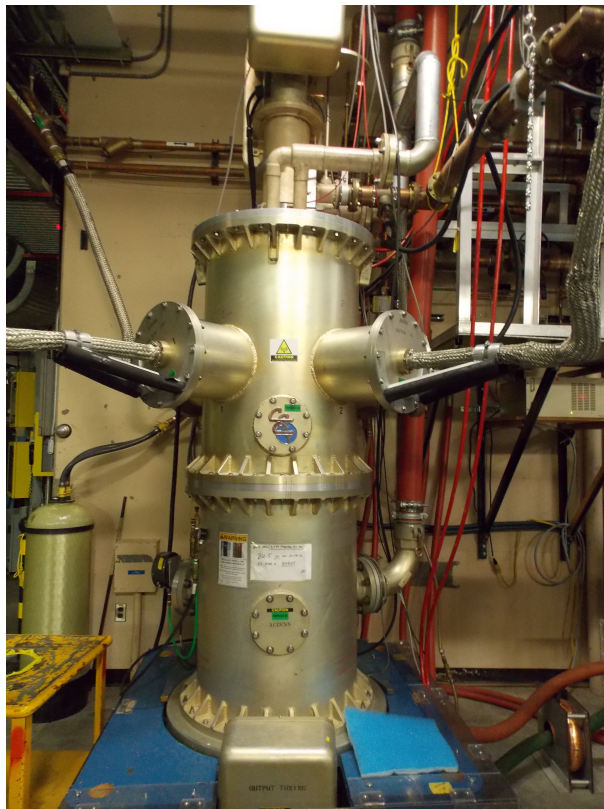
Figure 1.6: The LANSCE 201RF MHz triode FPA for DTL Module 1.
