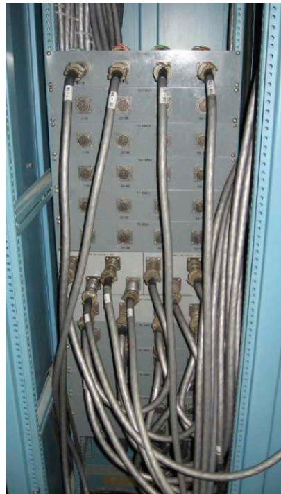
Slit and collector actuators
