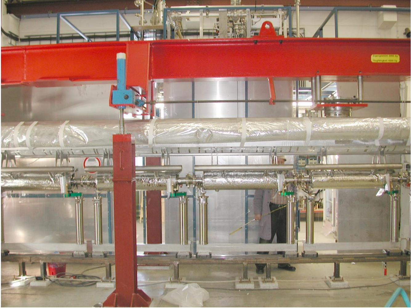
String in the assembly area
