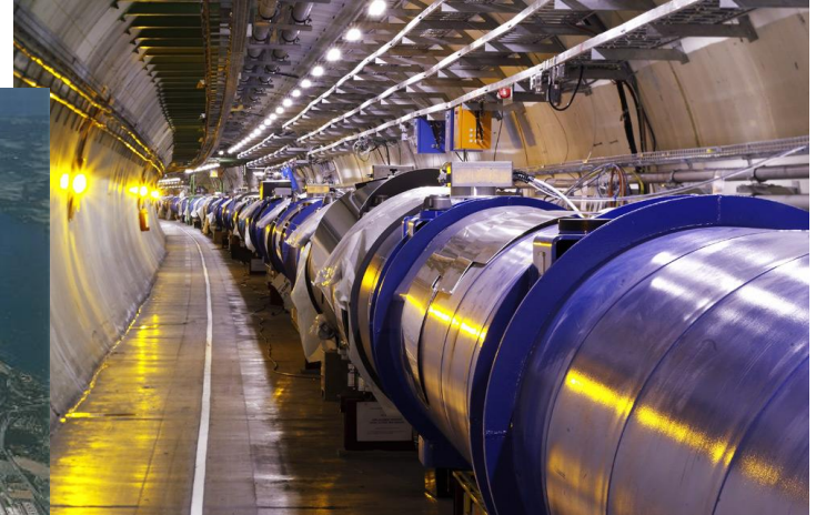
View inside the tunnel.
