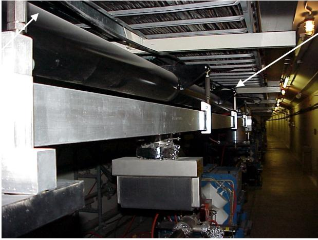
Struts adjust in Y-direction & Roll
